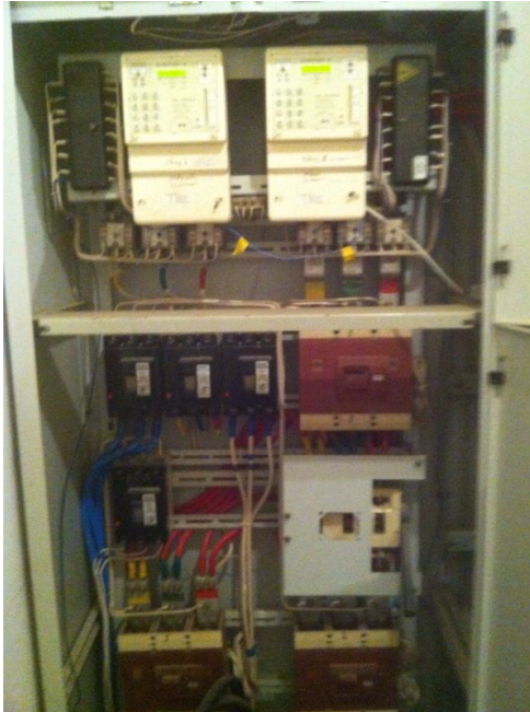
Figure 7.3: Incoming panel of the building
