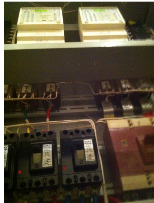
Figure 7.6: Input circuit breakers
