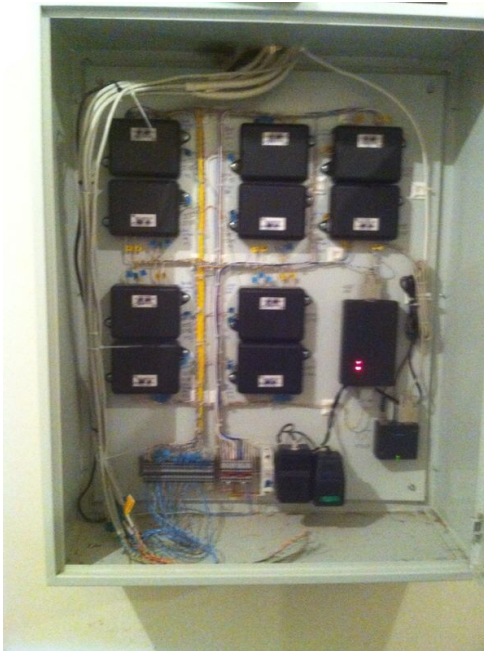
Figure 7.7: Panel with devices that gather and process information from meters and then transmits it via GSM modem
