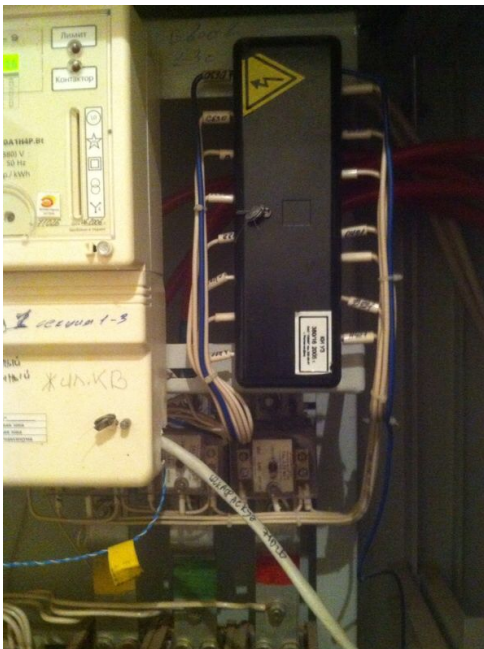
Figure 7.5: Terminal box
