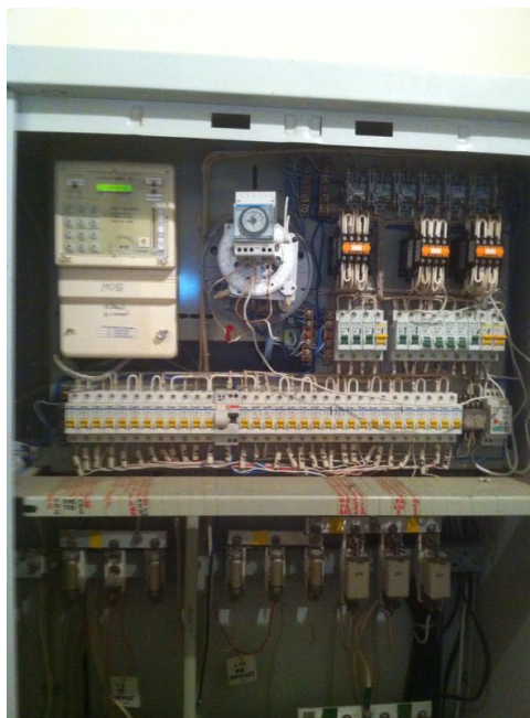
Figure 7.9: Panel for energy accounting of the common areas (elevators, water pump, etc)
