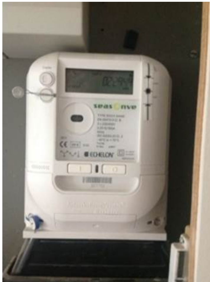
Figure 3.11: Echelon main meter.
